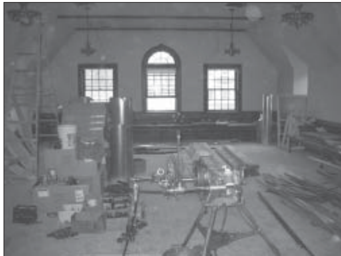
Hergenhan Recreation Center — Interior renovation work
