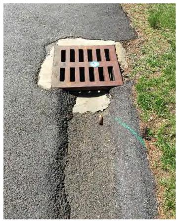
Deteriorated condition of stormwater drain limits function
