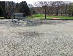
Parking lot in deteriorated condition; lack of striping does not allow for efficient parking.
