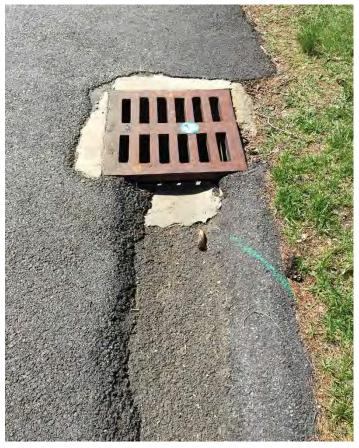
Deteriorated condition of stormwater drain limits function
