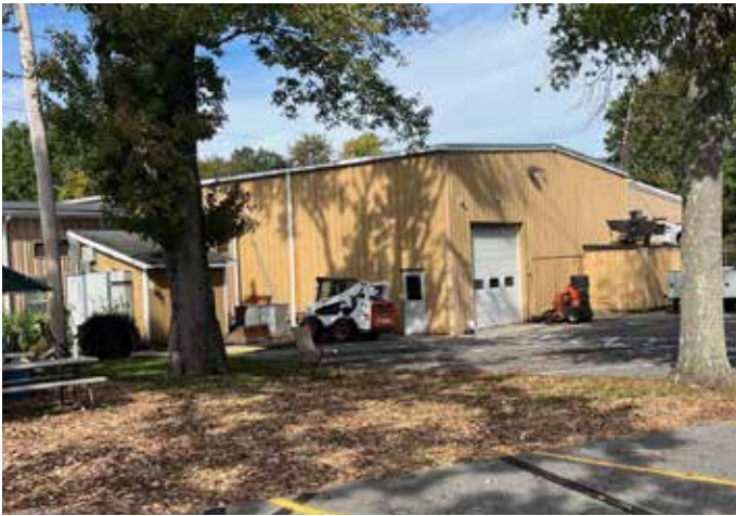
Existing Highway Garage Building
