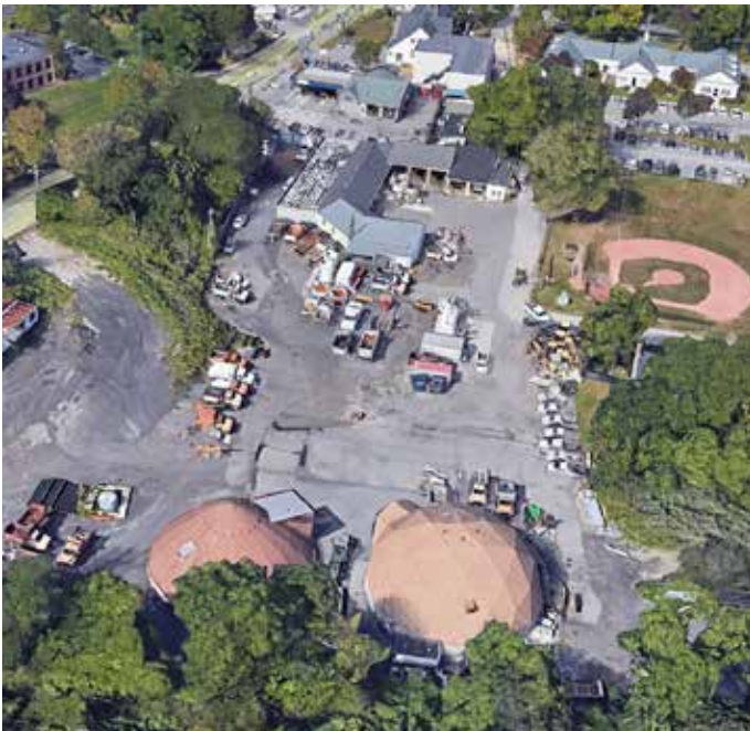
Existing Highway Garage Site
