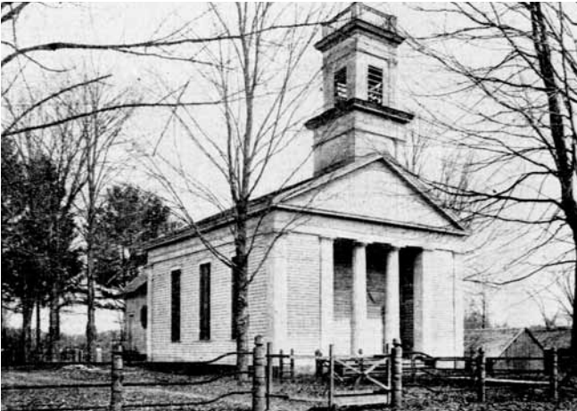
THE EPISCOPAL CHURCH OF ST. STEPHENS AT ARMONK Scheduled for Removal
