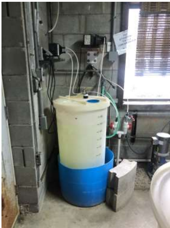
Photograph 17 - View of chlorination tank and feed system, facing south.
