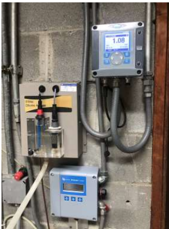
Photograph 18 - View of chlorine analyzer located in main pump room, facing west.
