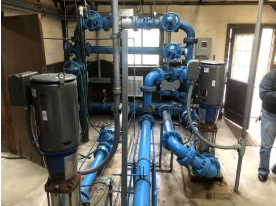
Photograph 13 - View of main pump house booster pumps and associated piping, facing south.
